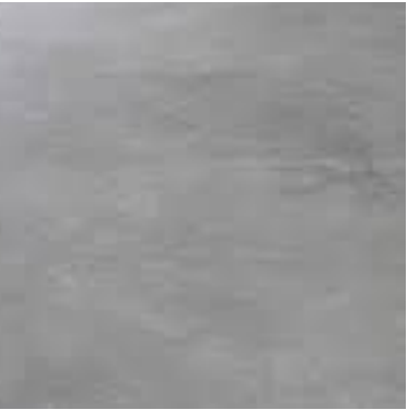
F-06 Concrete Finish Core, Structural walls, Basement level floors
