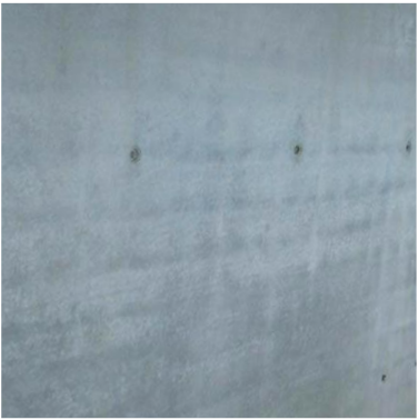
F-02 Off-Form Concrete Floor slab edge, Landscape walls
